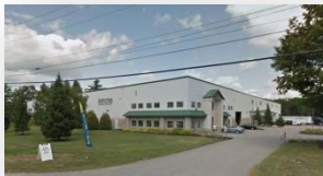
65 Spring Hill Road, Saco 40,000 SF Addition
