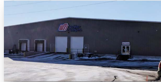
155 Rumery Road, South Portland Leased by Weber Fuel/Mattress Firm 47,040 SF
