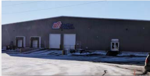
155 Rumery Road, South Portland 24,000 SF Spec Building
