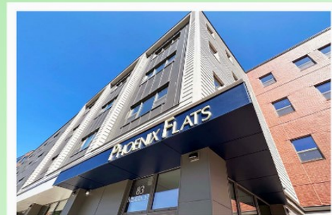
Phoenix Flats Photo courtesy of Community Housing of Maine
