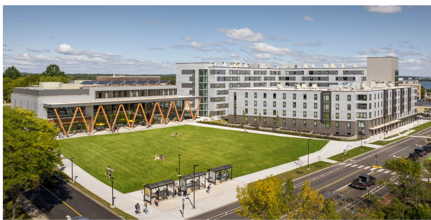
University of Southern Maine Portland Commons Residence Hall & McGoldrick Center for Career & Student Success Photo courtesy of Trent Bell Photography
