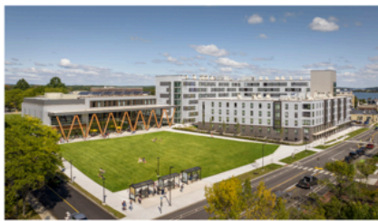
Photo courtesy of Trent Bell Photography
