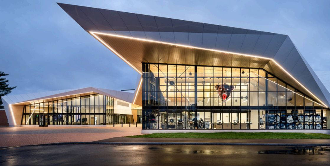
University of Maine Shawn Walsh Hockey Center and Harold Alfond Sports Arena Renovations and Additions Photo Credit: Ryan Bent
